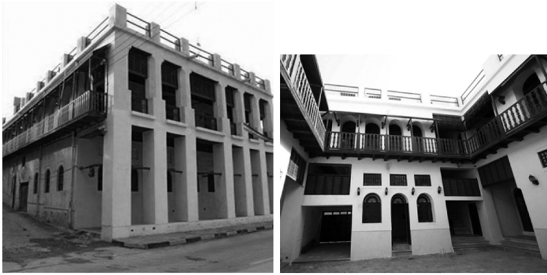
Figures 9-10. Taheri mansion exterior & interior courtyard views.
